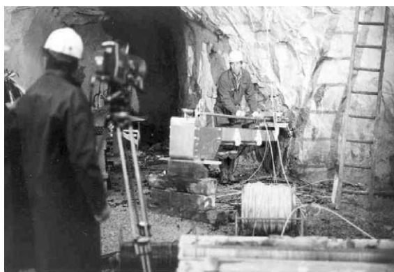
Fig. 1. Installation of in situ tests underground.
